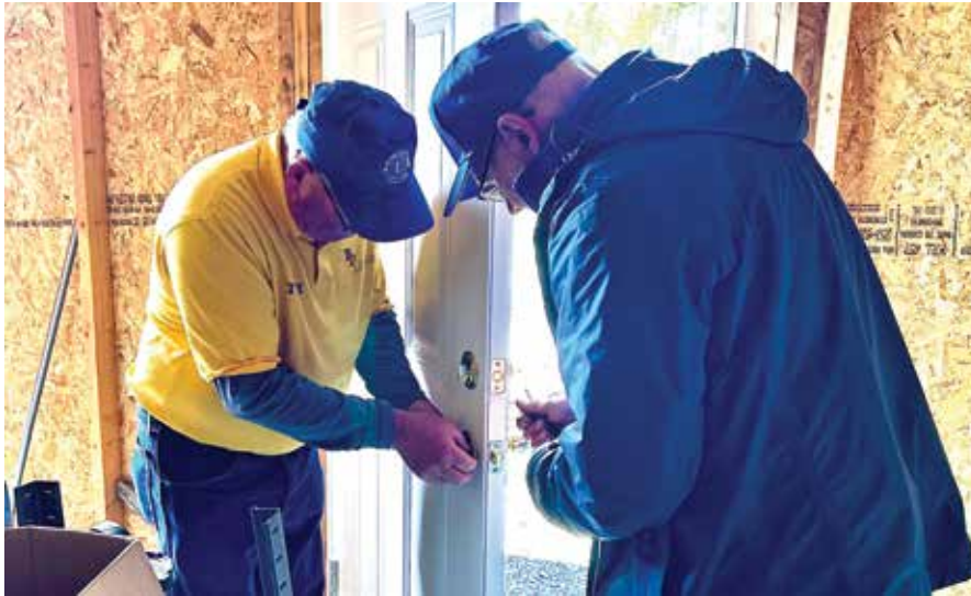
Broadalbin-Perth Lions Tom Kevlin, left, and Mike Auricchio, right, team up to install the locking hardware on one of the new doors on one of the structures at the Broadalbin Athletic Fields. The fields, also referred to as the "Field of Dreams", have been a longterm community service project of the Lions since 2008. (Photo courtesy Broadalbin-Perth Lions/Lion Valerie Kevlin).
